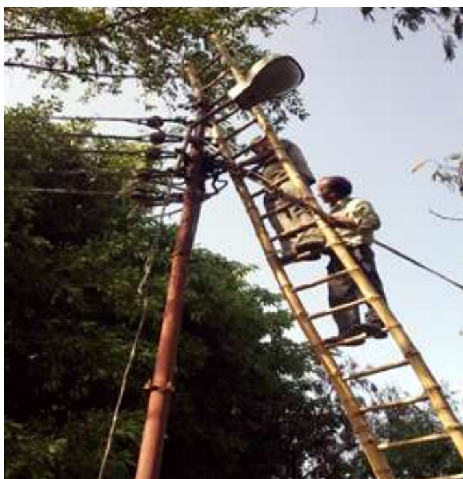
Providing and fixing of overhead line from marketing centre to the broiler farm
