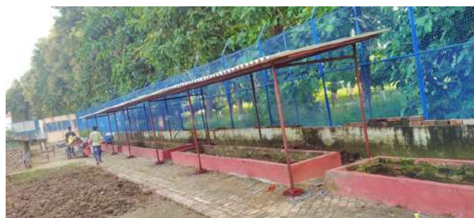
Renovation of sheds in the Giri Gram Takniki Park
